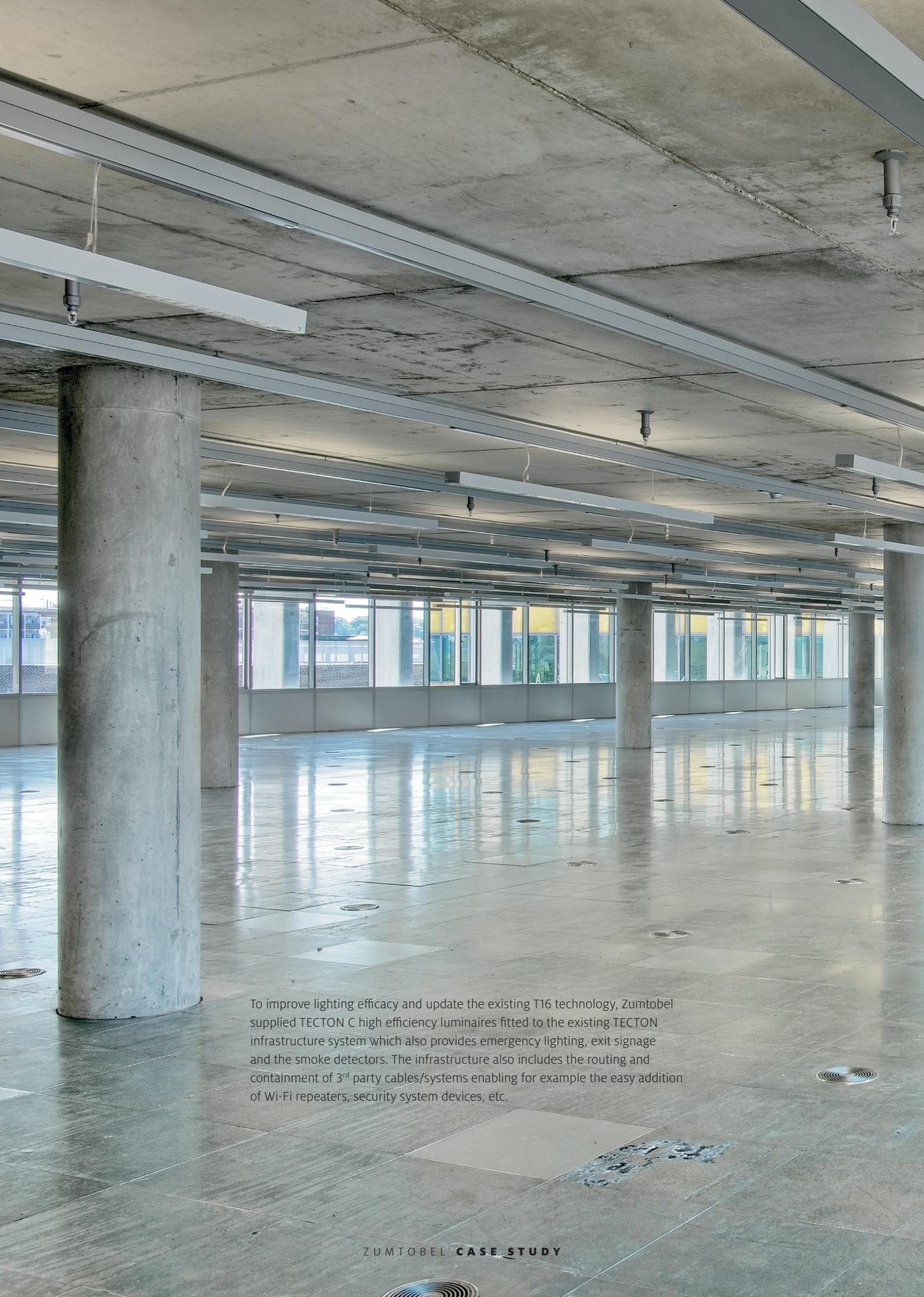
To improve lighting efficacy and update the existing T16 technology, Zumtobel supplied TECTON C high efficiency luminaires fitted to the existing TECTON infrastructure system which also provides emergency lighting, exit signage and the smoke detectors. The infrastructure also includes the routing and containment of 3<sup>rd</sup> party cables/systems enabling for example the easy addition of Wi-Fi repeaters, security system devices, etc.
