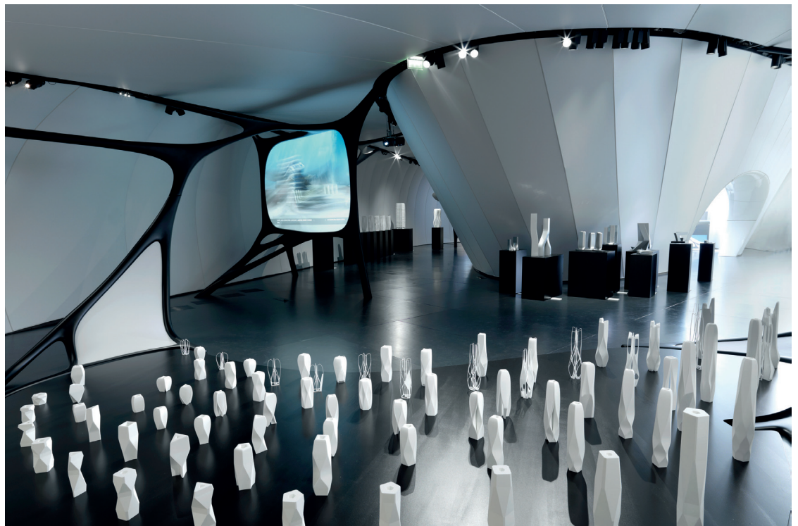
B3 | The lighting fixtures of the Arcos LED spotlight range and the Supersystem lighting system integrated into the black CNC milled guiding rails remain completely unobtrusive. The contrast between the light room segments – focussed on the exhibits – and the dark room segments cannot fail to attract the visitors' attention.
